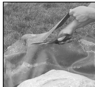
Trim off any excess liner.
